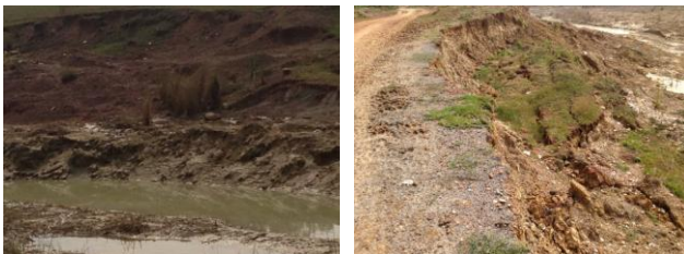
Figure 2 Severely Damaged Slopes
