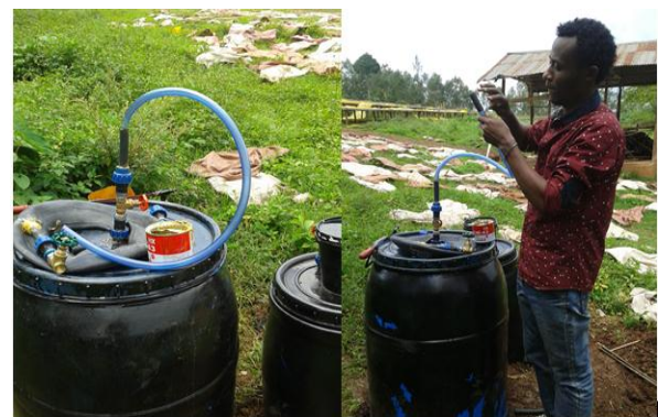
Figure 5: Bio gas digester construction for wet and dry coffee pulp
