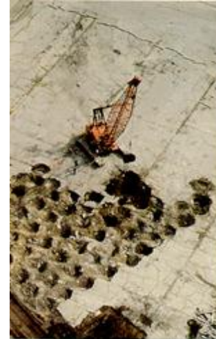
Fig.1 Dynamic Compaction
