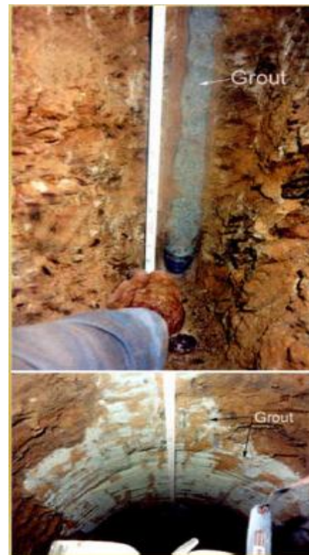
Fig.3 Compaction Grouting
