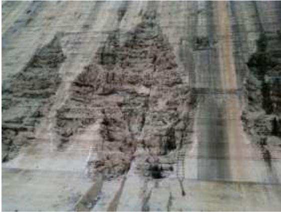
**Fig. 2 Cavitation Damage on Nagarjuna Sagar Dam.**
