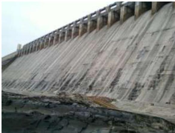
**Fig. 3 Erosion of Nagarjuna Sagar Spillway.**
