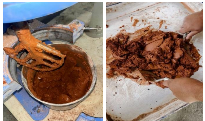
Figure 5: Mixing of Polymer-Modified Lime Mortar
