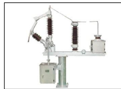
FIGURE 6 FIELD EXAMPLE OF A NEUTRAL POINT DEVICE
