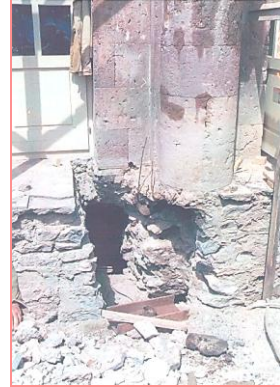
Figure 11. Temporary support under the existing arches (a) and the carved-out part of the foundation under the one quarter of the column section (b)
