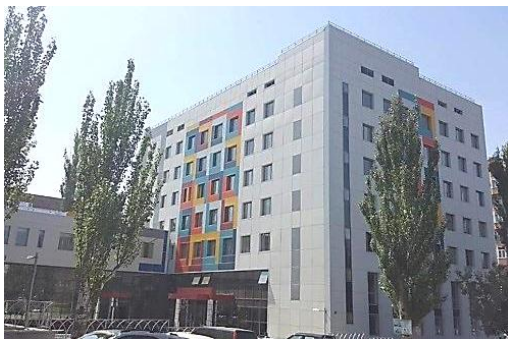
Figure 13. View of the existing 8-story R/C Hematology Center Hospital Building (HCHB) before (a) and after retrofitting by base isolation (b) with simultaneous renovation of the whole building
