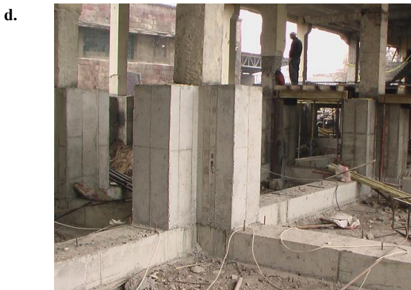
Figure 25. (Continued) eismic isolators' lower sockets installed before casting the columns' concrete (c); final view of the new columns constructed around the existing columns (d)
