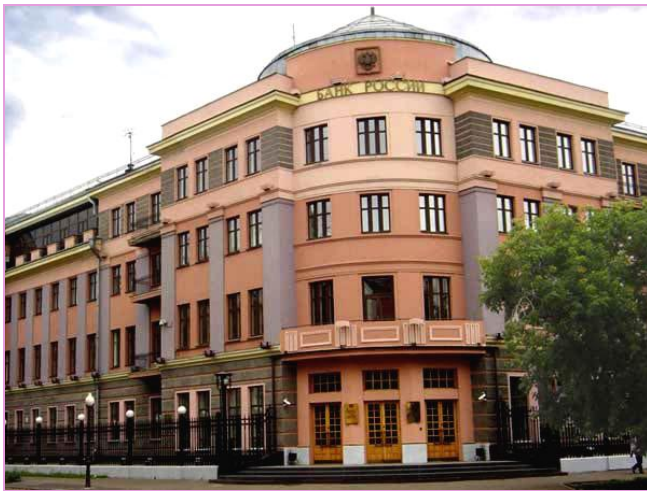
Figure 27. View of the bank building retrofitted by base isolation in the city of Irkutsk
