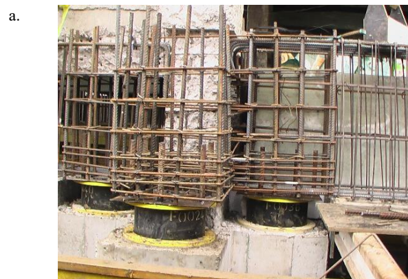
Figure 25. (Continued) eismic isolators' lower sockets installed before casting the columns' concrete (c); final view of the new columns constructed around the existing columns (d)
