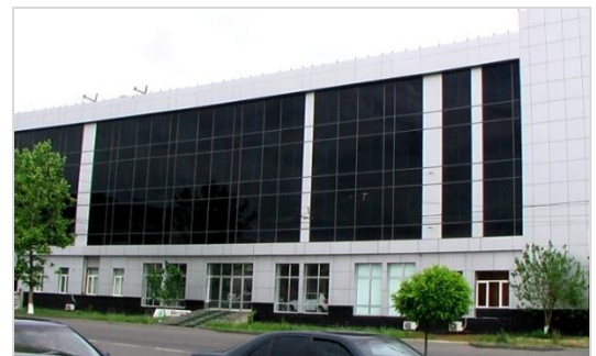
Figure 23. View of the existing 4-story industrial R/C frame building before (a) and after retrofitting by base isolation (b) with simultaneous renovation of the whole building
