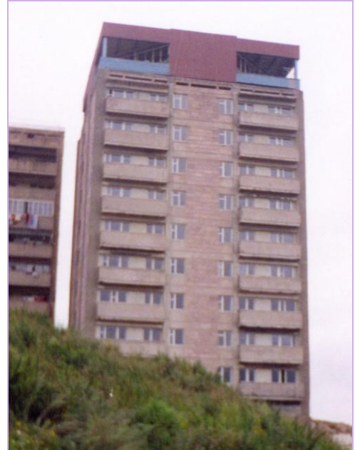
Figure 6. General views of the two existing R/C frame 9-story apartment buildings protected by AIUF in Vanadzor
