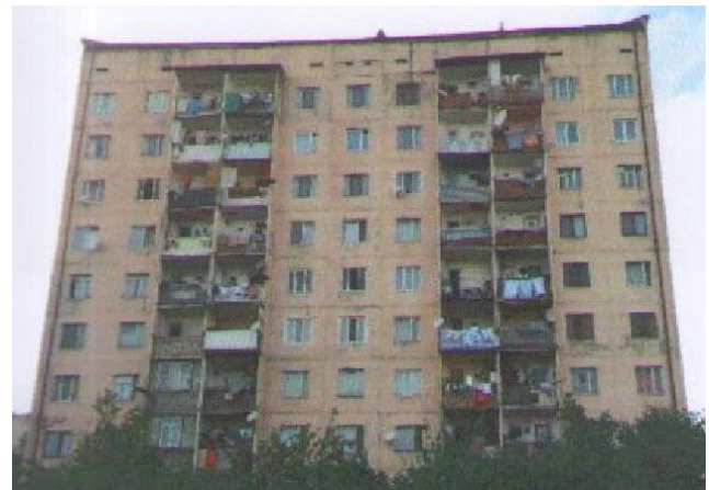
Figure 30. View of the existing 9-story large-panel apartment building retrofitted by base isolation in Azerbaijan
