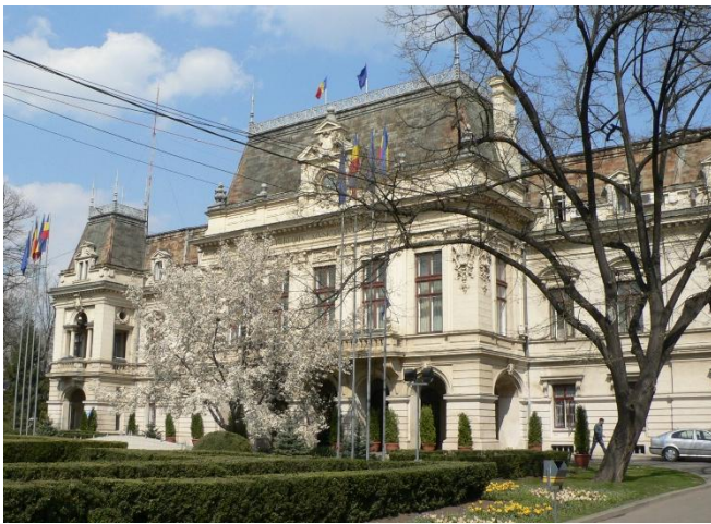
Figure 37. View of the 2-story Iasi City Hall building with stone bearing walls
