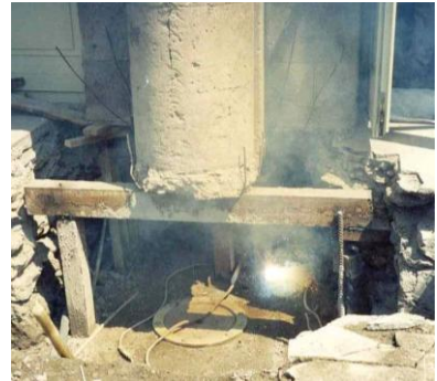
Figure 11. Temporary support under the existing arches (a) and the carved-out part of the foundation under the one quarter of the column section (b)
