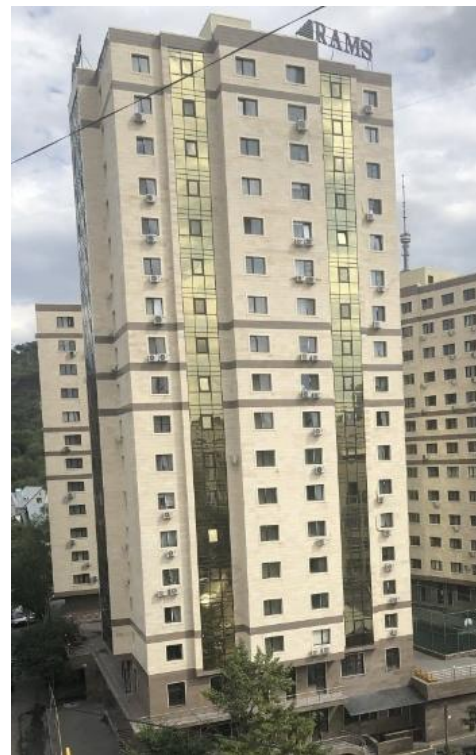
Figure 41. View of the existing 19-story (including two basement floors) apartment building located on the Dostyk ave. 138 in the city of Almaty to be retrofitted by base isolation
