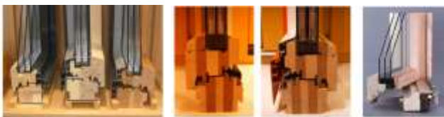
Fig. 22 Triple layered windows that are specific for passive houses
