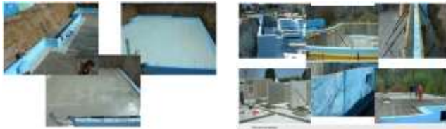
Fig. 21 Thermal insulation with extruded polystyrene under the foundation
